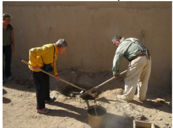
DJ helping "Jose" in making adobe bricks.
