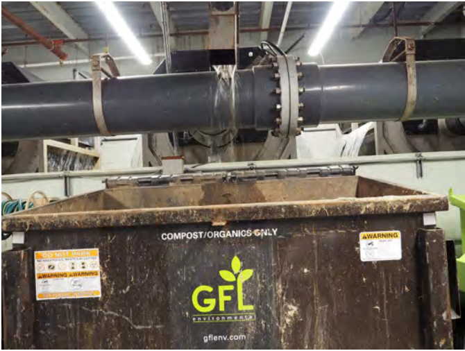
Solid waste filtered from hippo pool going into bin for composting (from IE tour in November)
