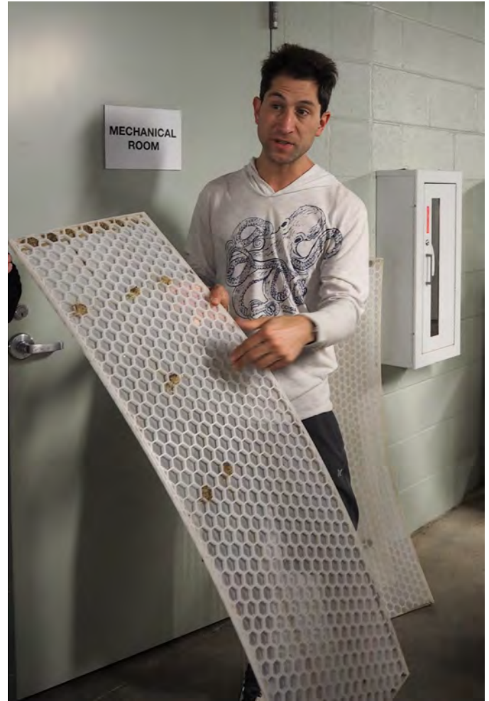
One of honeycomb sediment filters, the mesh micron size determines efficiency of waste material removed from water (from IE tour in November)
